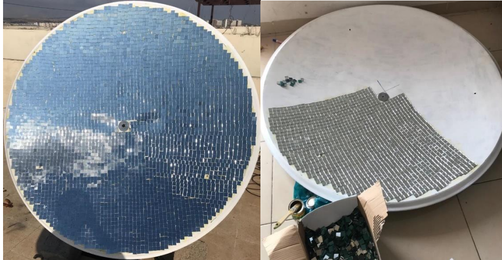
Figure 3.3 Solar collector with mirrors ben installed
