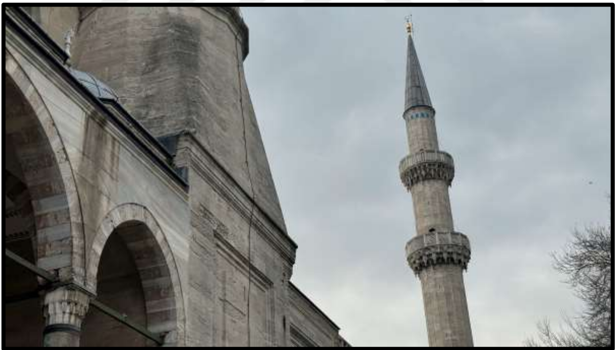
Figure 3.35: Exterior Details of Suleymaniye Mosque Captured by Author.
