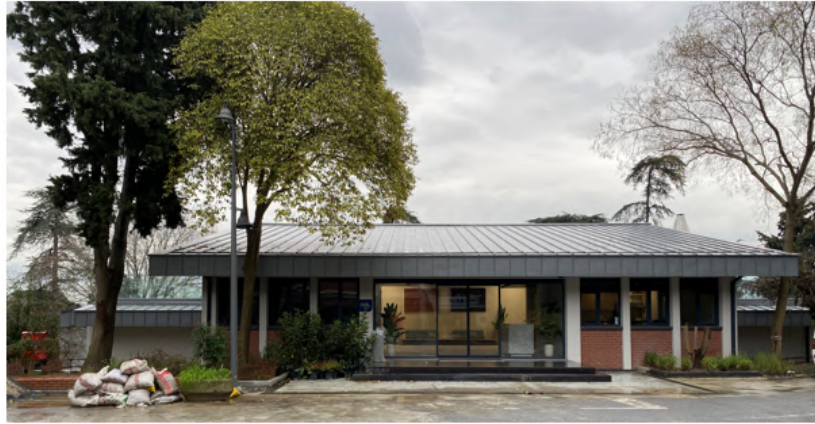
Figure 3.7. Data science and artificial intelligence institute building from front.
