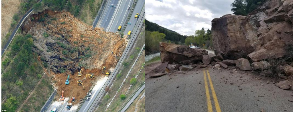
Figure 2.1 Example of Landslide and Rockfall
