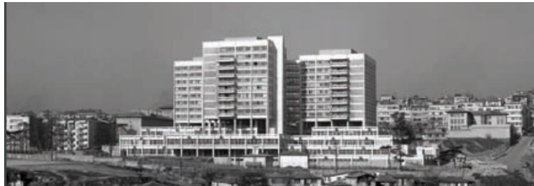
Figure 3.36 Front View, Şişli Children's Hospital
