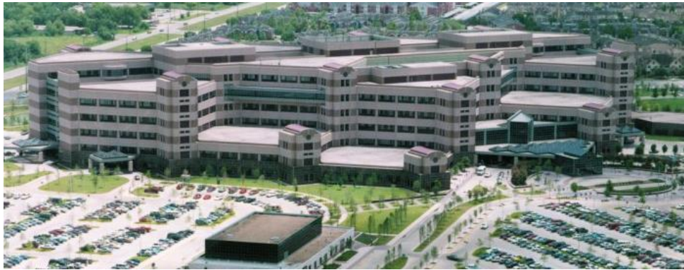
Figure 2.28 Veterans Administration Medical Center in Houston
