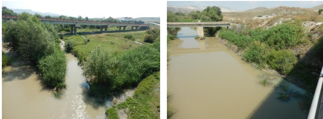
Figure 4.14. The current riverbed, banks and floodplain conditions of the target location E12A045 and its upstream – Images taken in between December 2017 and August 2018
