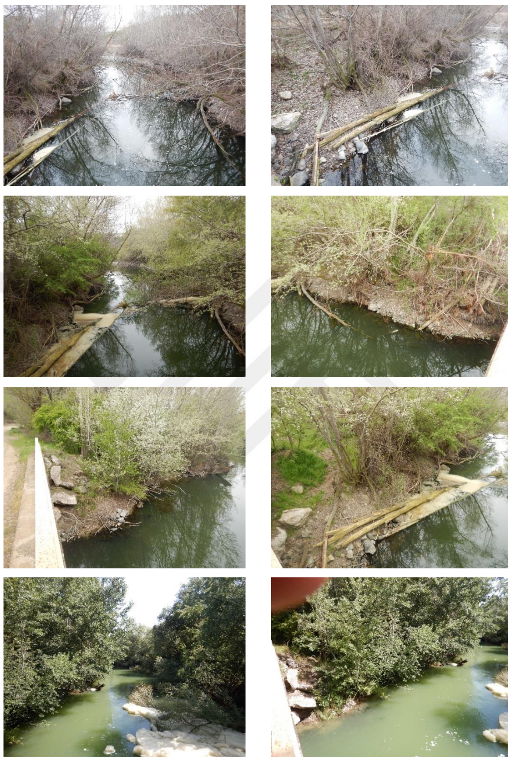
Figure 4.16. The current riverbed, banks and floodplain conditions of the target location D12A034 and its upstream – Images taken in between December 2017 and August 2018
