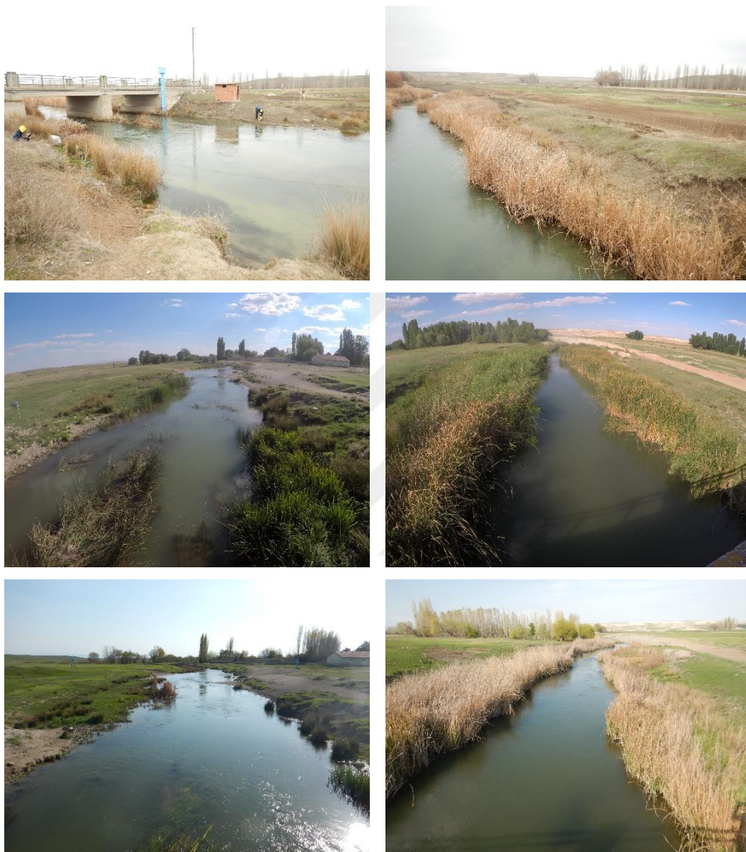
Figure 4.12. The current riverbed, banks and floodplain conditions of the target location E12A024 and its upstream – Images taken in between December 2017 and August 2018
