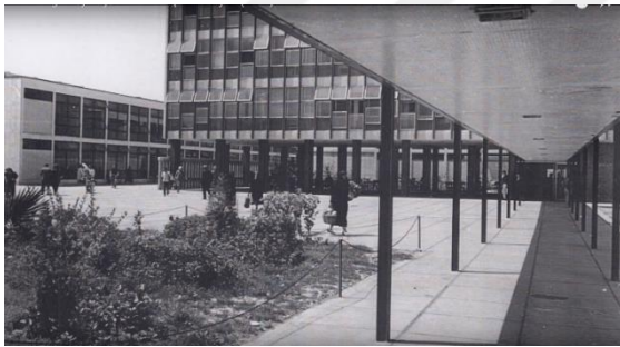
Fig.4.22: Sakarya Government House inner courtyard, 1960s.
