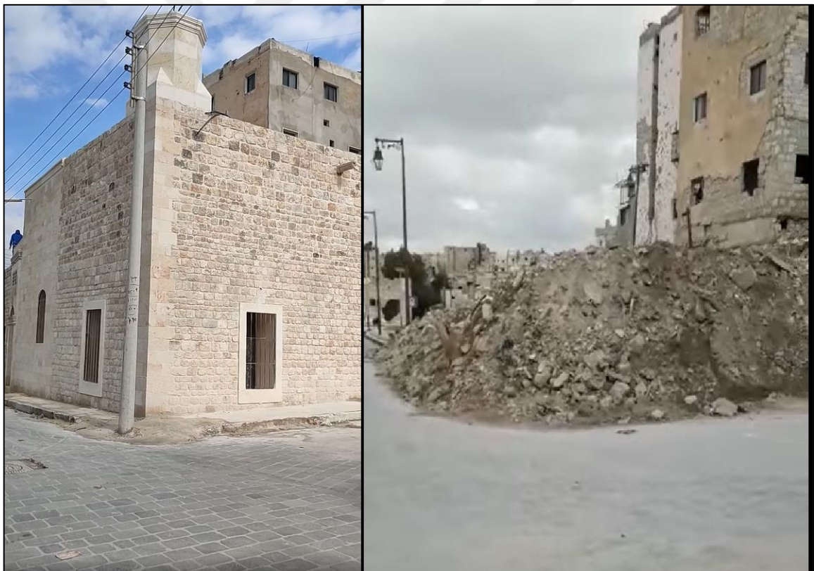
Figure 6.8. Rebuilding a mosque in Aleppo by local community, photo by Salem Ahmad, 2022.
