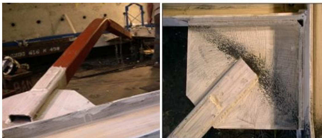
a) Brace buckling deformation
