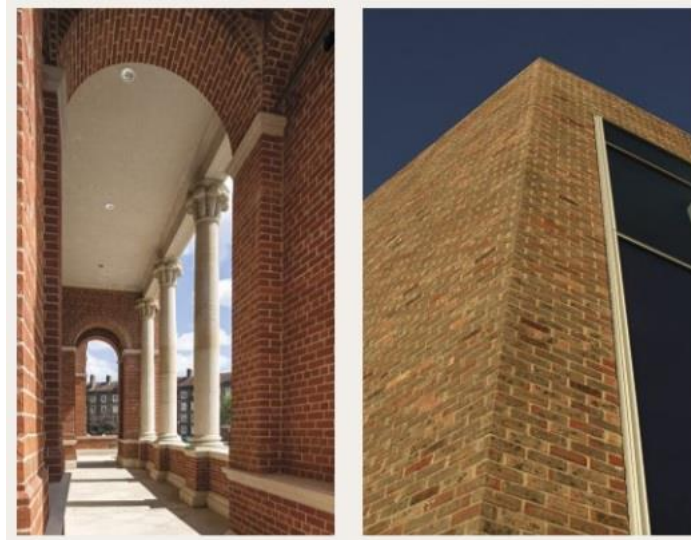
Figure 2.1 Brick structures (Ibstock, 2016)
