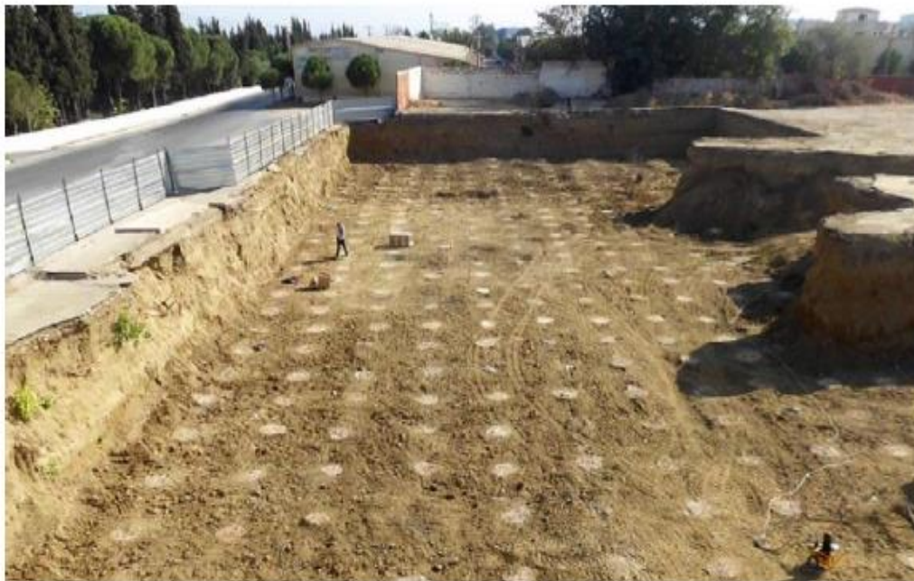
Figure 2.13 Top view of lime column application
