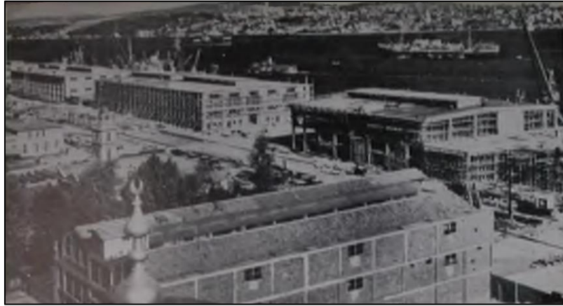
Figure 3.43. Construction of the Warehouse and Docks in the Salıpazarı Port [148].
