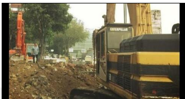
Figure 3.69. Construction machinery started to demolish in Gezi Park [281].
