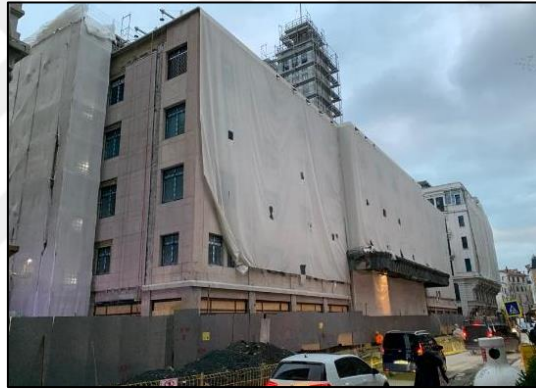
Figure 3.89. The view of Karaköy Passenger Hall, which is under renovation, photo taken by author.
