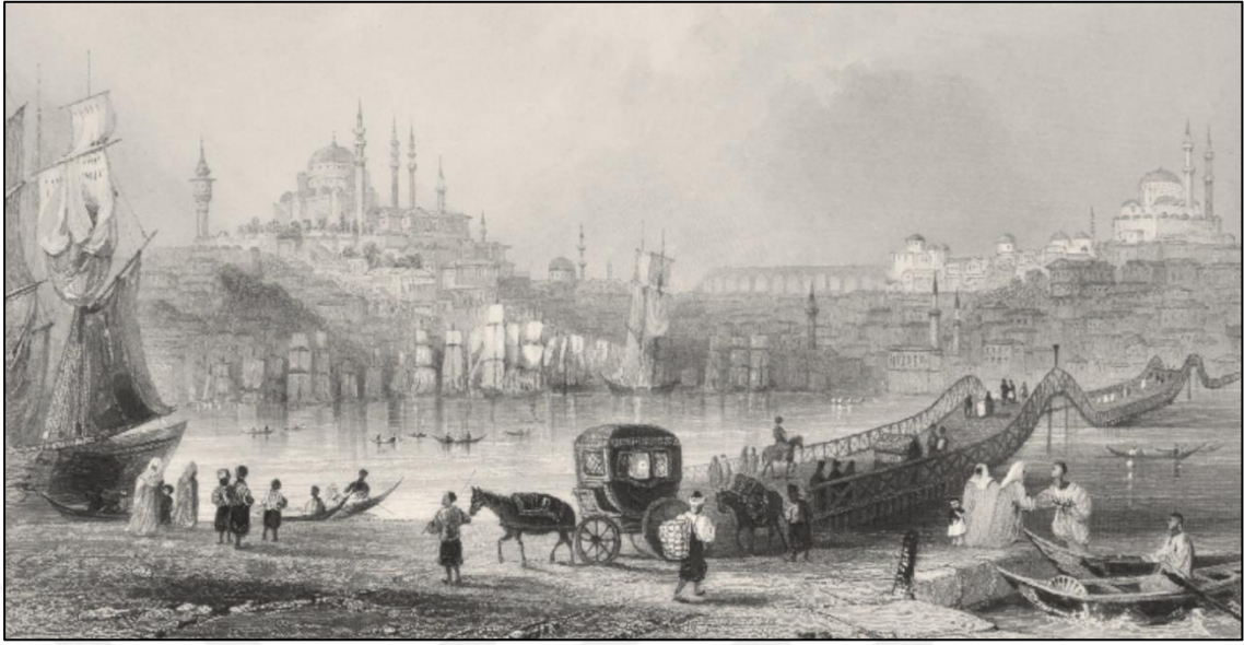
Figure 3.4. Cisir-i Cedid Bridge, built by Sultan II. Mahmut in 1836 [50].
