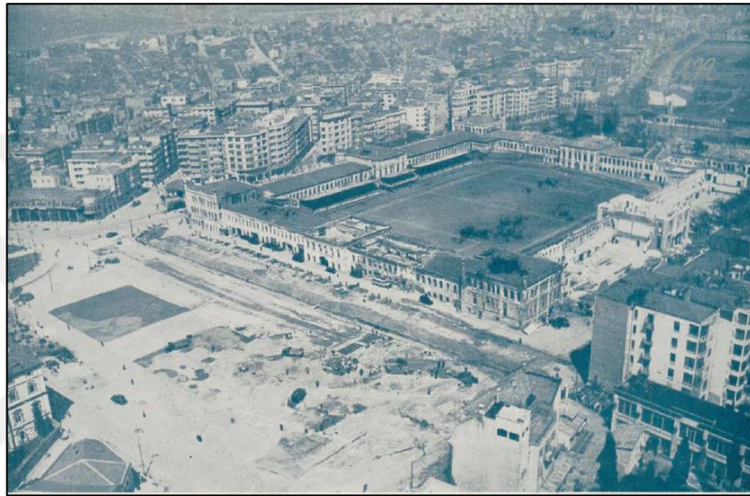
Figure 3.21. Artillery Barracks demolished as part of Gezi Park construction [112].
