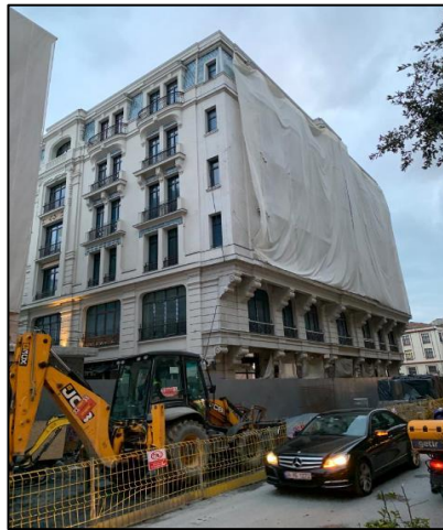
Figure 3.90. The view of Merkez Han, which is under renovation, from Kemankeş Street, photo taken by author.
