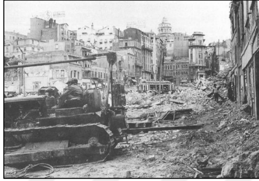
Figure 3.35. The demolition works in Karaköy Square dated 1958 [157].
