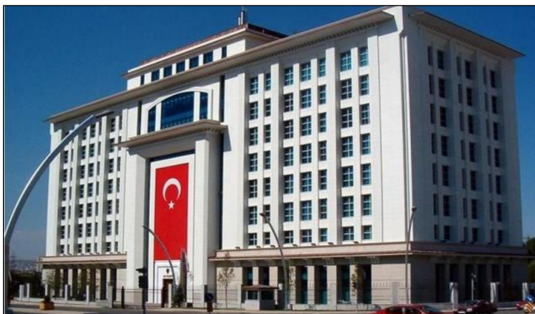
Figure 3.78. The AK Party Headquarters, where the effects of the Ottoman-Seljuk architectural style can be observed [293].
