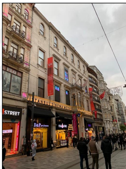
Figure 3.76. View of renewed Atlas Cinema (İstanbul Cinema Museum) from İstiklal Street, photo taken by author.
