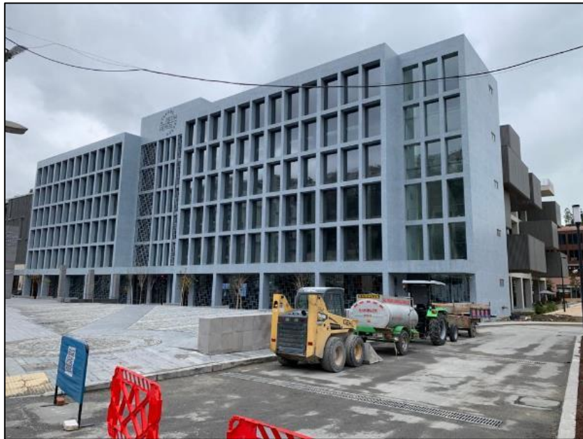
Figure 3.96. Entrance façade of İRHM facing Meclis-i Mebusan Street, photo taken by author.
