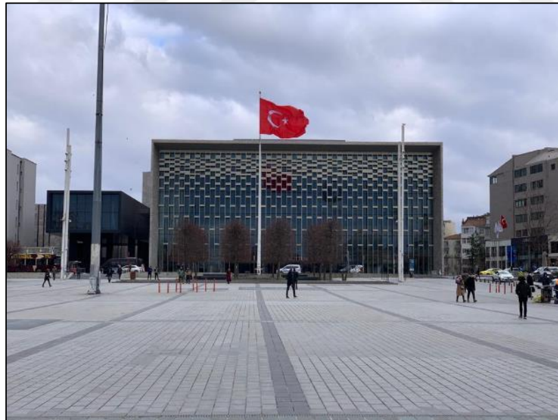
Figure 3.80. View of AKM from Taksim Square, photo taken by author.
