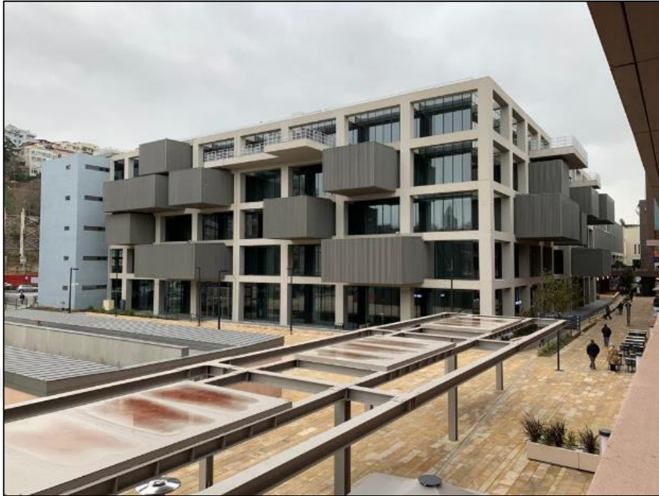
Figure 4.7 İRHM's reinforced concrete carcass facade and cantilevered container units, photo taken by author.
