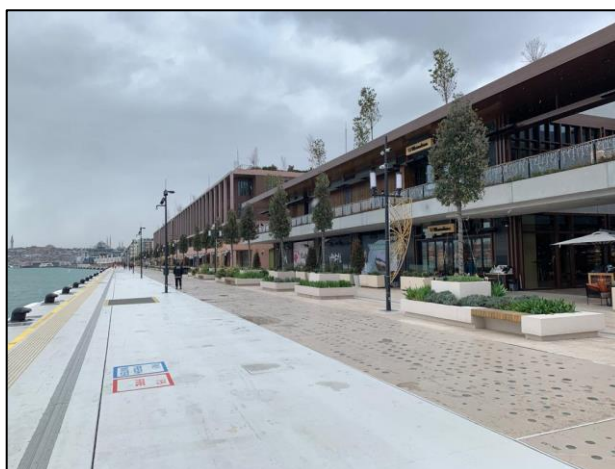
Figure 3.83. The coastline that opens to the public with a modular (opening and closing) cover system, photo taken by author.
