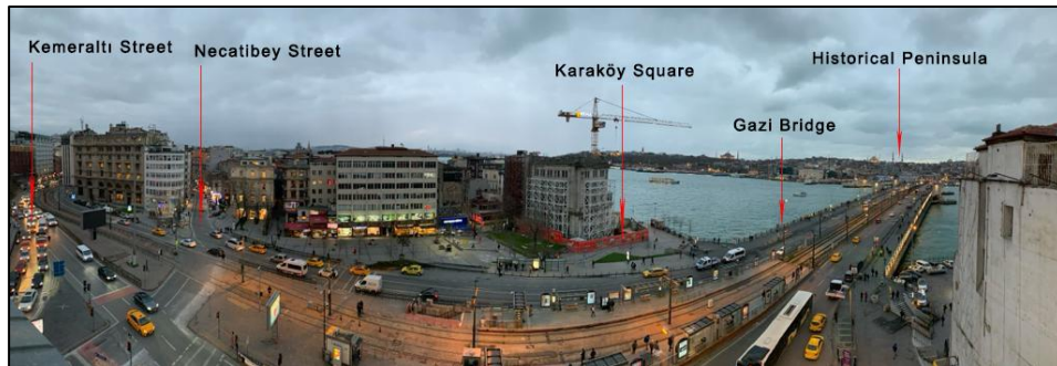
Figure 3.40. The current state of Karaköy Square and Gazi Bridge, photo taken by author.
