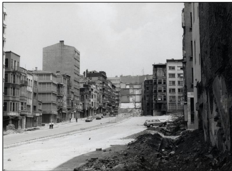
Figure 3.54. Demolition of Tarlabası Boulevard in 1988 [210].
