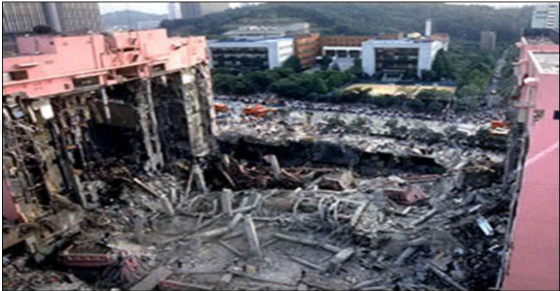
Figure 1.2 Post-collapse photograph of the Sampoong Department Store (Gardner et. al. 2002)
