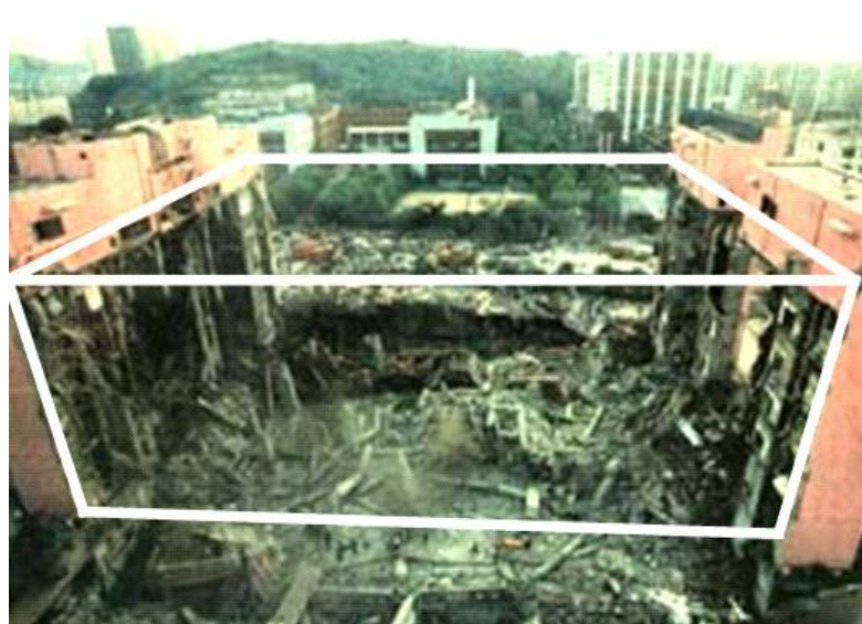
Figure 2.1 Sampoong department store collapse (Gardner et. al. 2002).
