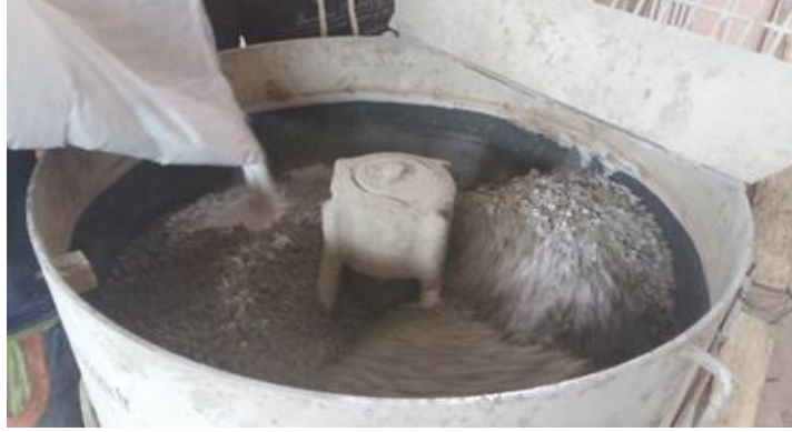
Figure 3.7 mixing for normal concrete.
