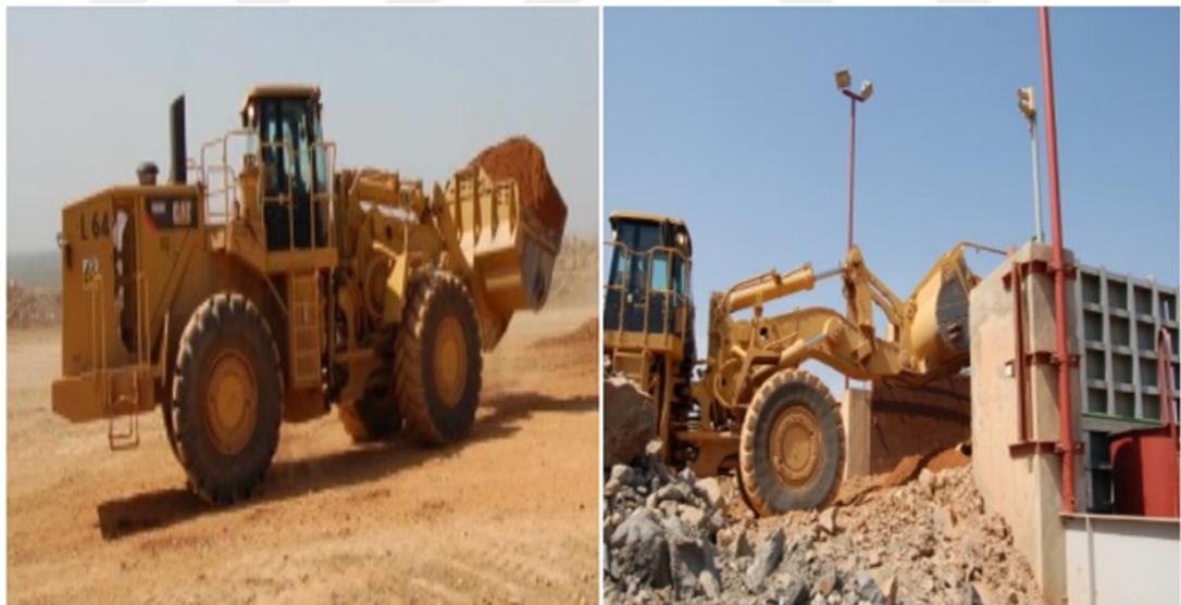
Figure 3.13 Loader ROM pad and Feeding crusher (Personal archive, 2017)
