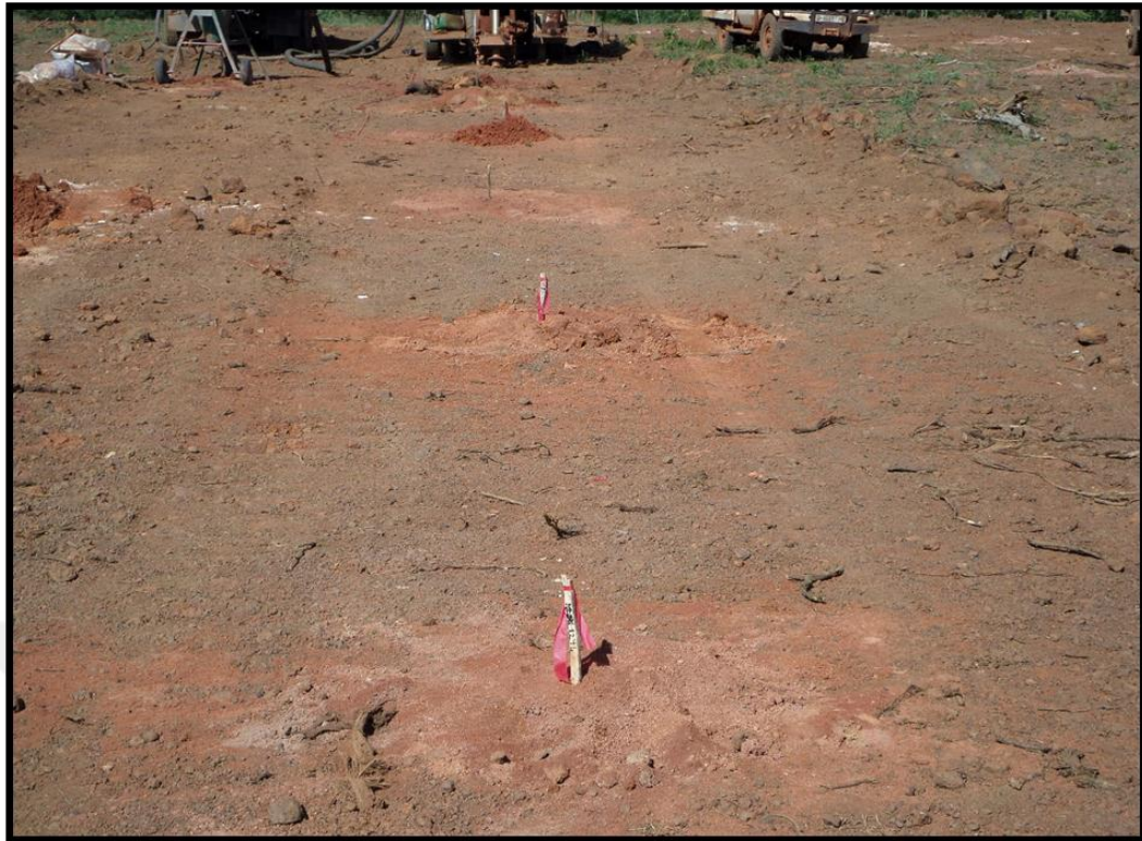
Figure 3.6 GC holes back filled and re-pegged (Personal archive, 2017)
