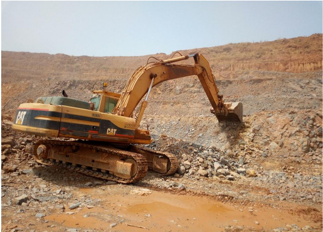
Figure 3.9 Bulldozer cleanup wall (Personal archive, 2017)
