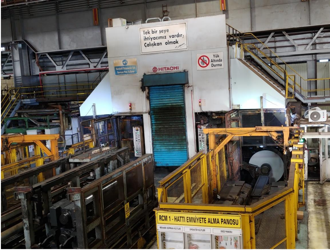
Figure 3.3. Borçelik cold rolling mill line.
