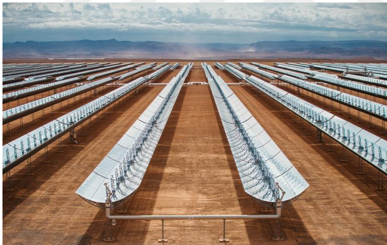
Figure 1.1. An image from Noor 1 CSP plant [3]
