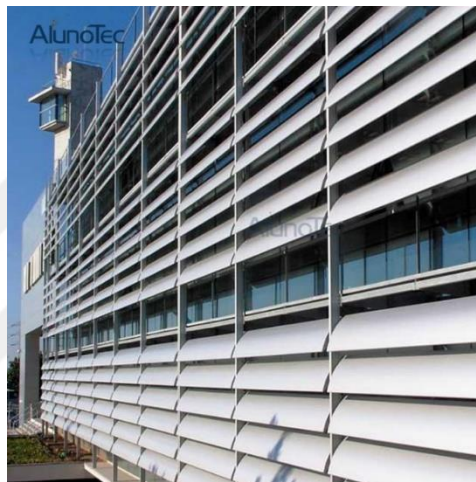
Figure 3.2: Horizontal slat solar shades [66].
