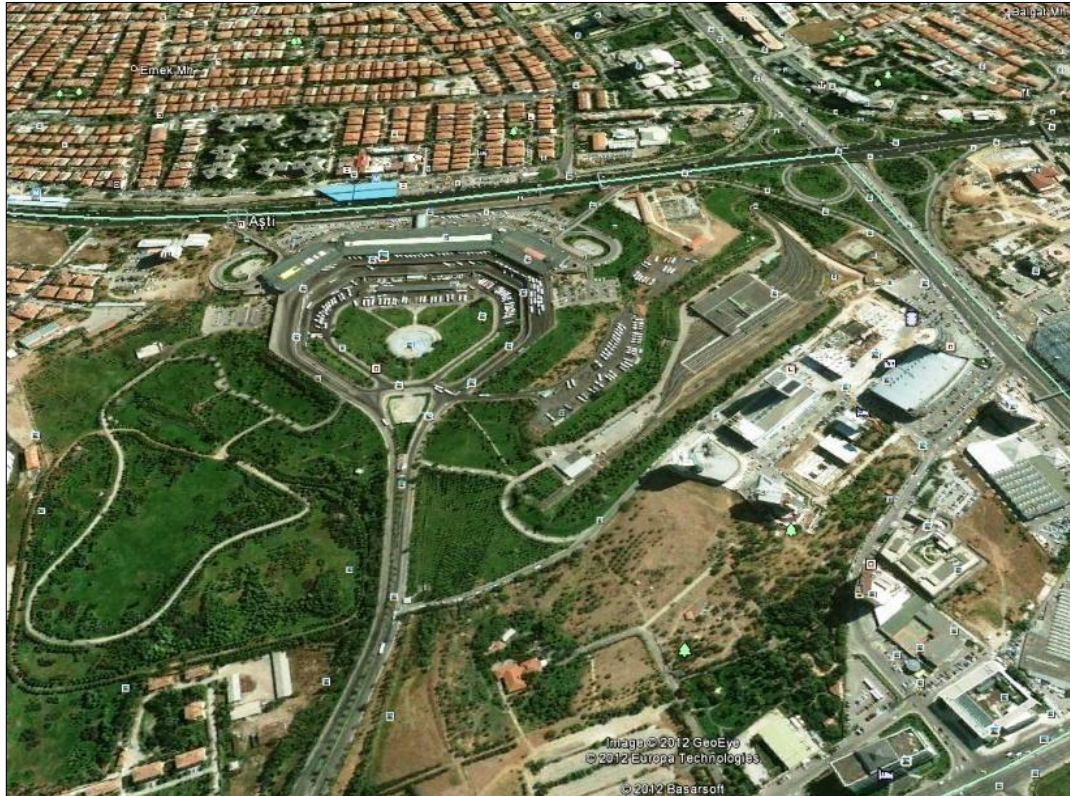
Figure 2: ASTI Terminal Complex Aerial View (Source: http://www.1yenimesajinizvar.com/wp-content/uploads/2012/10/kusbakisi-asti.jpg )
