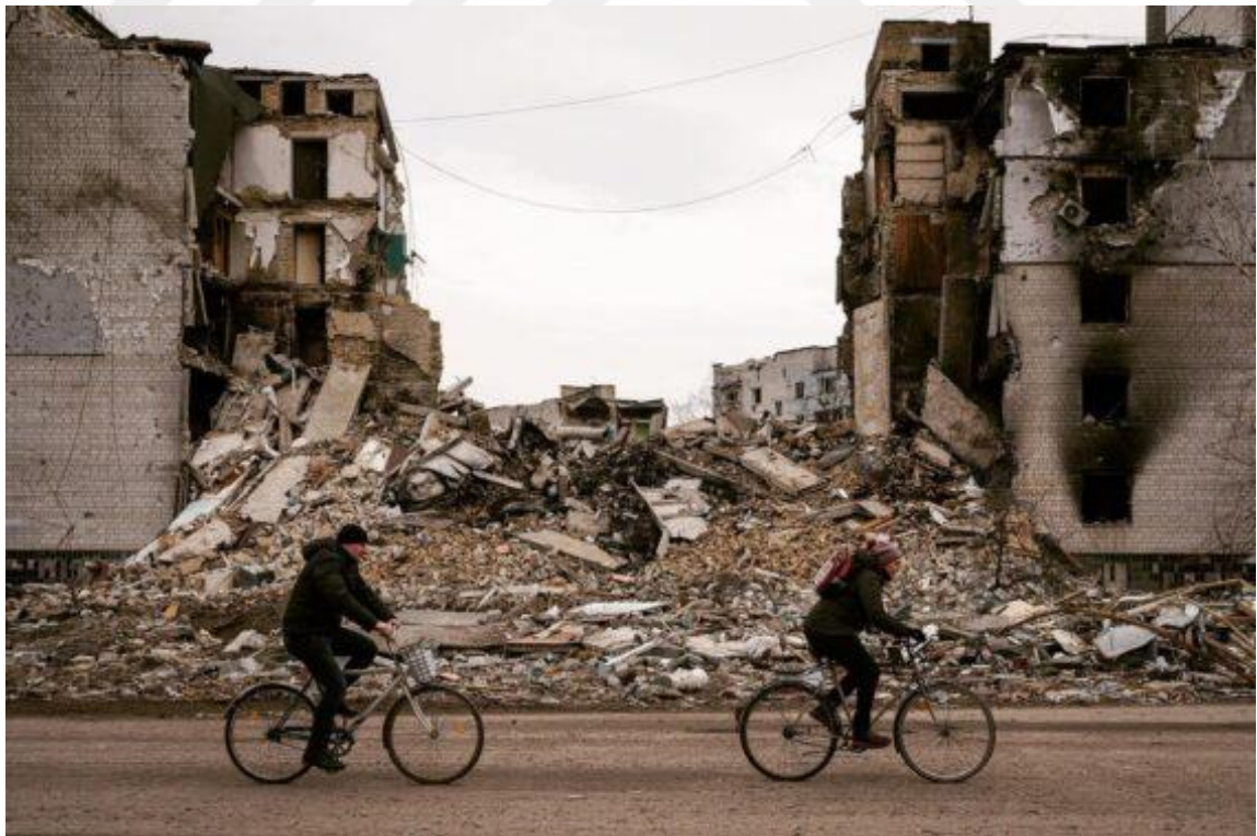
Figure 41. Destroyed buildings in the city of Borodyanka near Kyiv on the 6 th of April 2022 by the heavy Russian's army bombardments
