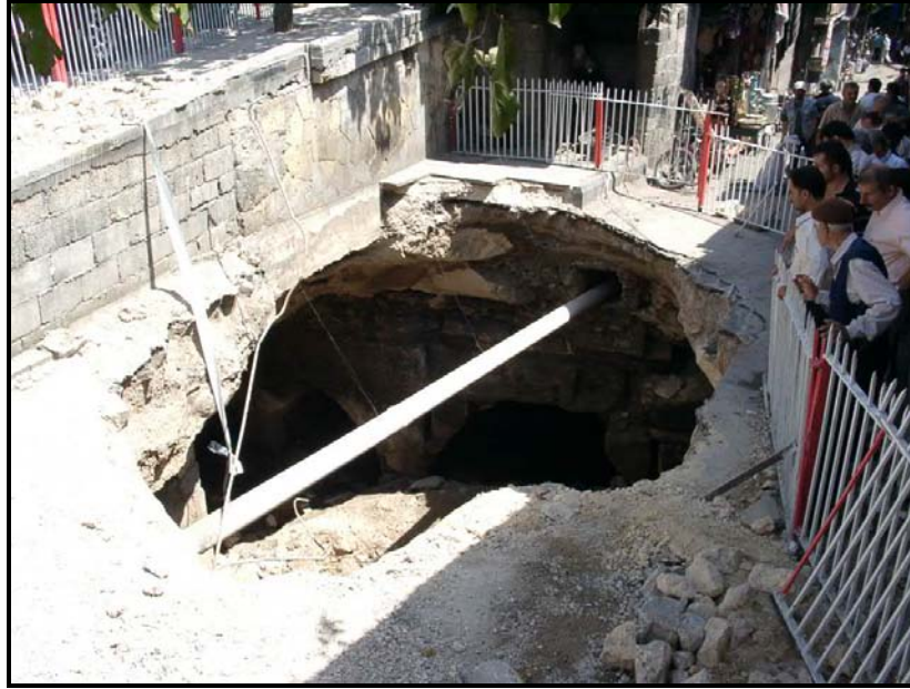
Figure 2.1. One of the collapsed caves at Hamdi Kutlar Street in Gaziantep
