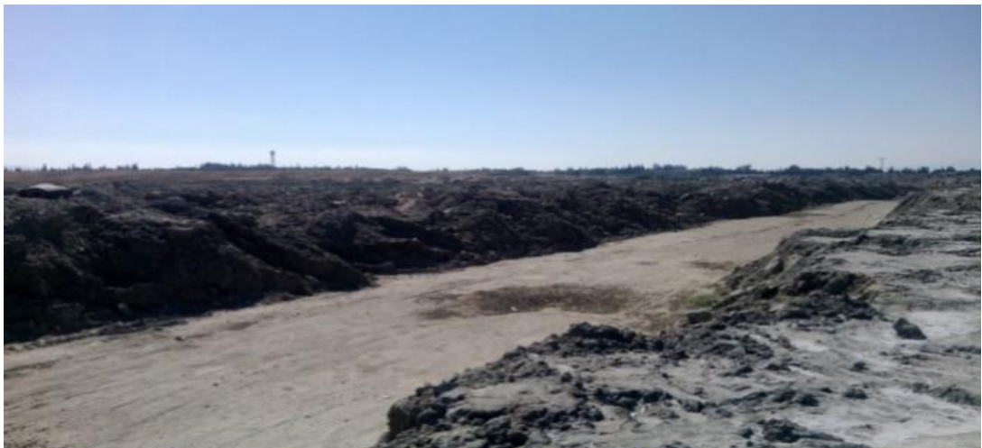
Figure 2.4 Site conditions (Personal archive, 2018)
