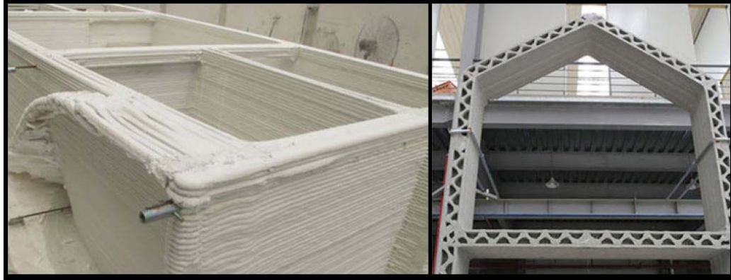
Figure 36. Partial rapid-prototyped house construction detail (Reinhardt, Saunders, & Burry, 2016, p. 96).
