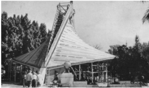
Figure 13. An exemplary hyperboloid surface under construction by Candela (Pedreschi, 2008, p. 16).
