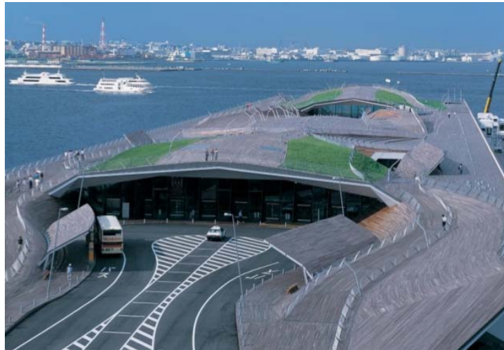
Figure 40. Yokohama International Port Terminal in Yokohama, Japan (Groenendijk & Vollaard, 2009, p. 140).
