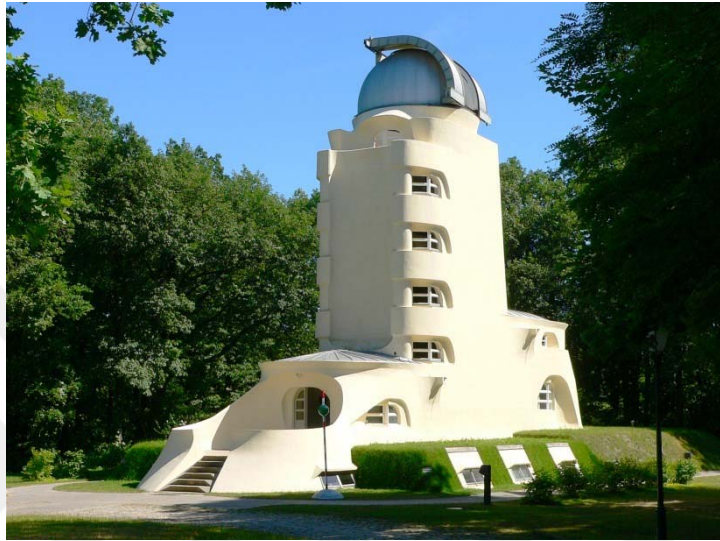
Figure 18. Einstein Tower in Potsdam, Germany (Weston, 2004, p. 44).
