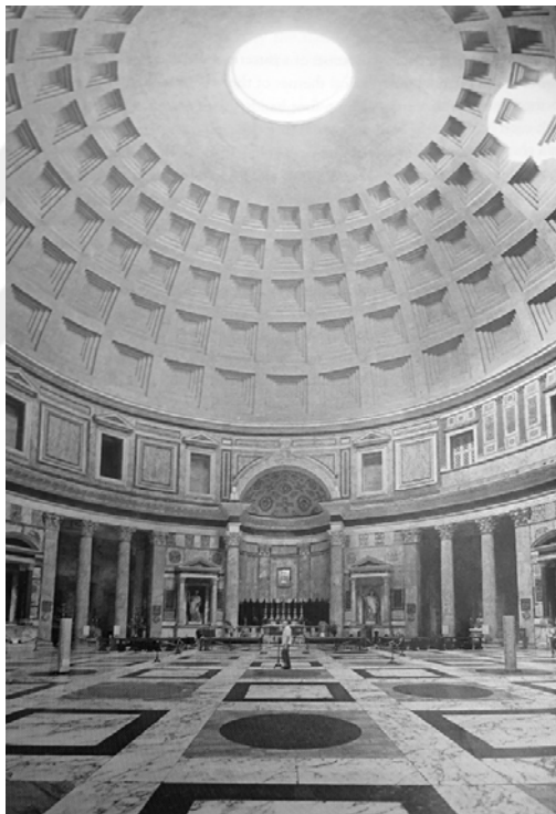
Figure 5. Pantheon interior view (Marder & Jones, 2015, p. 18).
