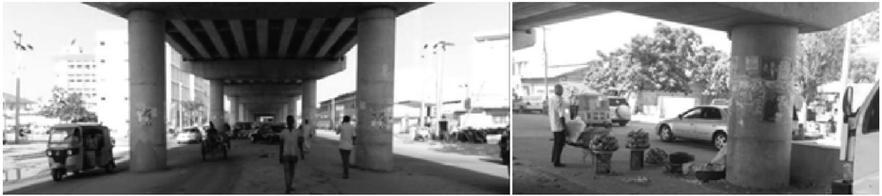
Figure 5.13: Structure of the street under the bridge at MM-Way. (Author, 2017).
