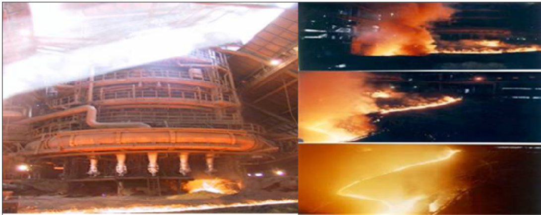
Figure 2.4 A general view of the Blast Furnace. Photograph of a blast furnace at the end of a tap with the mud gun in position at the taphole. The taphole drill is retracted and ready to be swung into position for use for the next tap (Isdemir, 2010).
