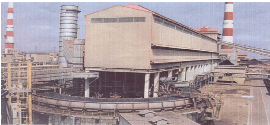
Figure 5.5 Induced draft rotary or circular sinter coolers, shown in process of construction (Poveromo, 1999).
