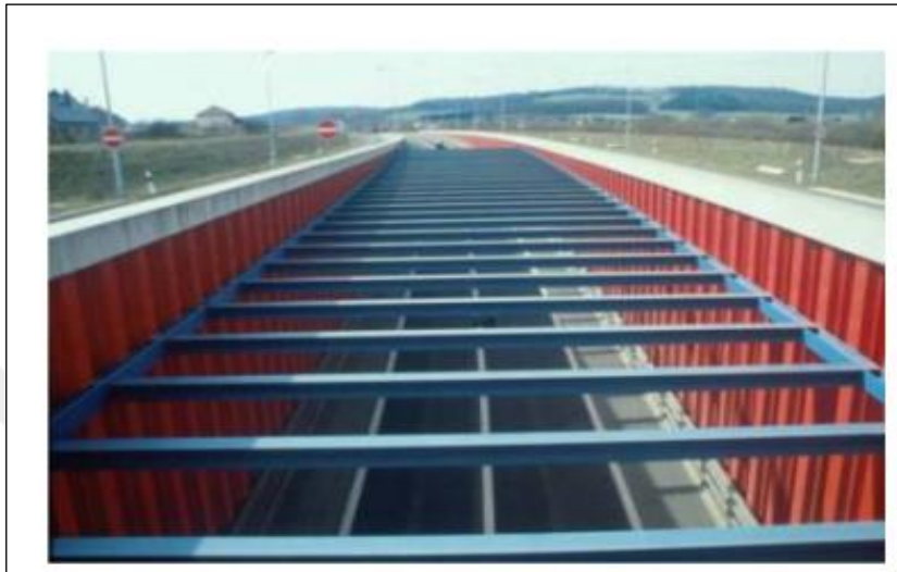
Figure 2.10: Sheet Pile Wall for Tunnel.[29]
