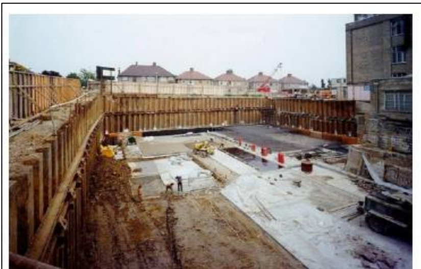
Figure 2.11: Anchored Sheet Pile Wall for Excavation Shoring.[29]
