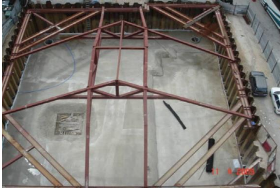
Figure 2.15: Lateral Support System. [85]
