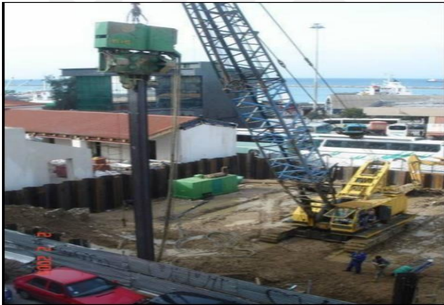
Figure 2.16: Vibratory Sheet Pile Driver. [85]
