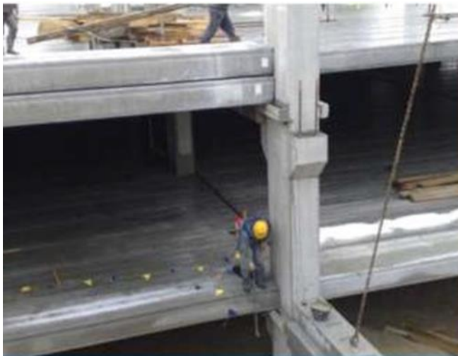
Figure 2.6: A dowel Connection Between a Beam and a Column.
