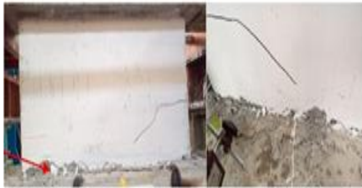
Figure 3.3: Observed Failure of Specimens with SS Failure.
