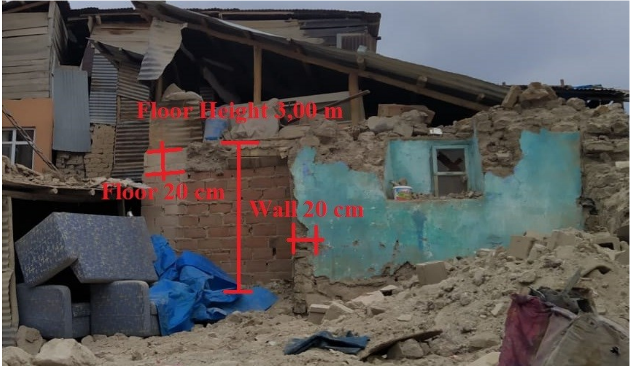
Figure 4.8 2nd stage demolition works in Sürsürü
