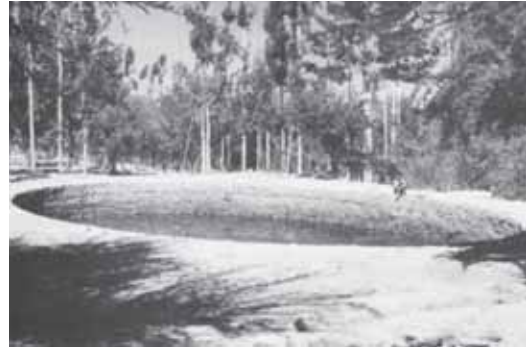
Figure 12. The water collection pool for distribution system at the Qanat's outlet in Pishkuh-i Yazd [10].
