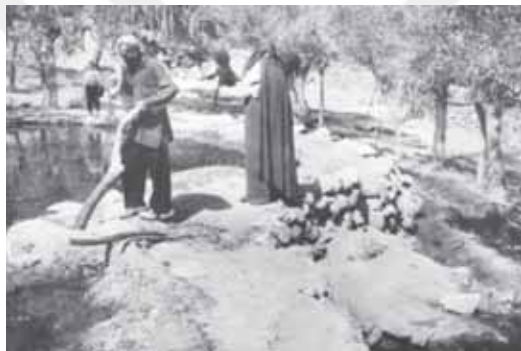
Figure 13. The water collection pool for distribution system at the Qanat's outlet [10].
