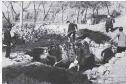
Figure 14. The cleaning process of the water collection pool at the Qanat's outlet in Pishkuh-i Yazd [10].
