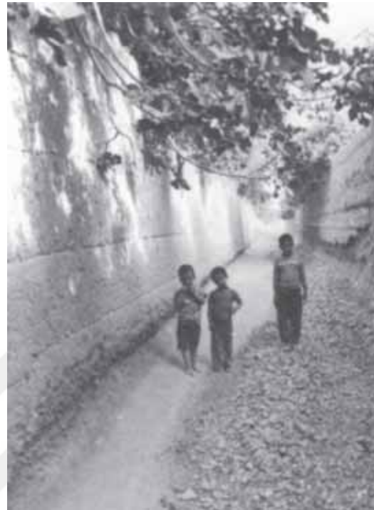
Figure 29. The erosion of walls by irrigation channel in Mehriz [9].
