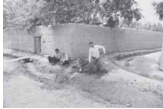
Figure 25. Diverting water from main irrigation channel into walled agricultural fields and orchards in Mehriz [9].
