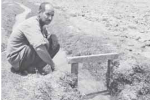
Figure 30. The wooden tool to measure the flow of water within water channels in Sar-i Yazd [10].
