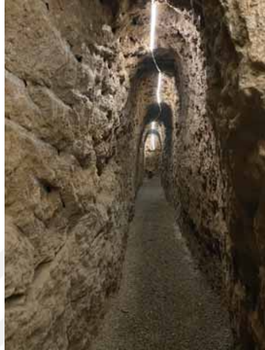
Figure 118. The water inlet to the private Payab . Photo by author in November 2023.
