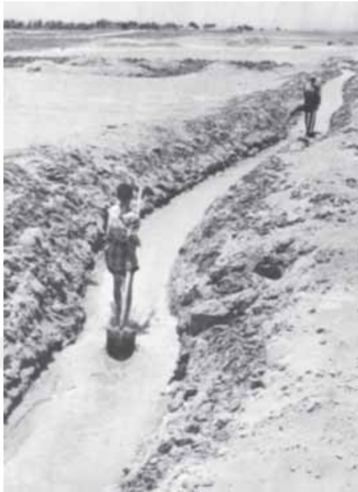
Figure 32. Dragging shovels in the water channels to move water and minimize leakage [10].
