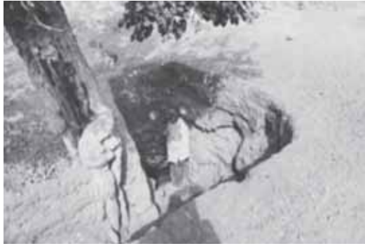
Figure 11. The Qanat's outlet ( Mazhar ) in Mehriz . The excavation is unusual, most outlets are at the surface [10].
