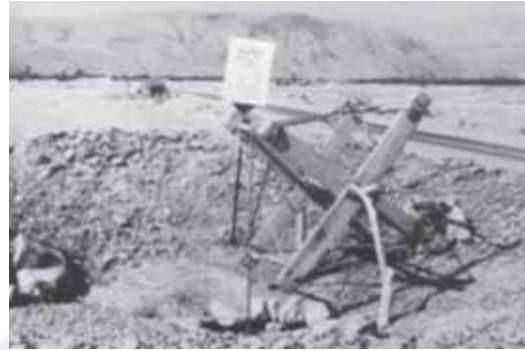
Figure 9. The windlass for lifting out the excavated materials and ventilation [10].
