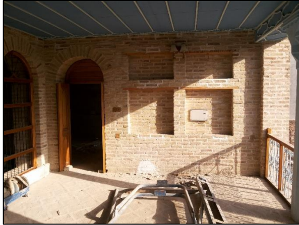
Figure 4.43. The Iwan doors of Osman Chawash house during restoration studies, photograph taken by author.
