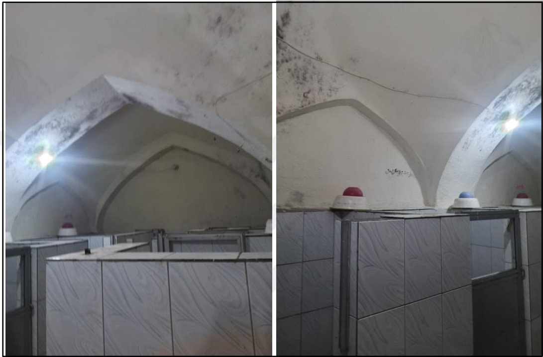
Figure 4.70. The separated bathes roof of Saiwan Hamam, photograph taken by author.
