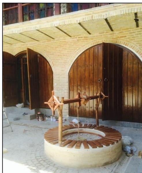
Figure 4.32. Shops of the Farah Hotel after Restoration 2021, photograph taken by author.
