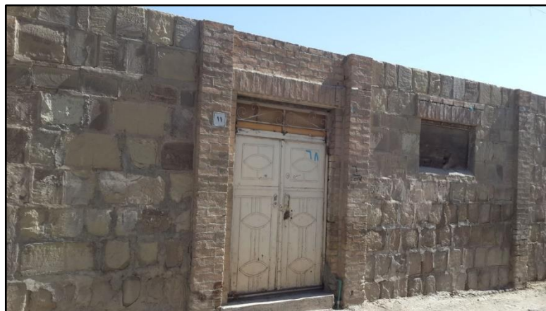
Figure 3.26. Wall built by Malkandi Stone, photograph taken by author.
