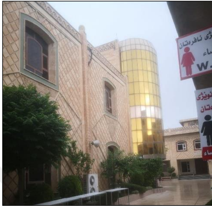
Figure 4.20 Renovated courtyard of Khanaqa mosque, photograph taken by author.
