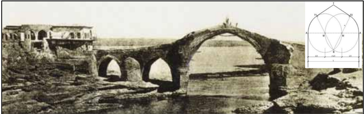
Figure 2.7. The Altunköprü Nâhiye – The oldest photograph of the Great Bridge in Kerkuk pointed arches can be seen in this old photo [Anonym].
