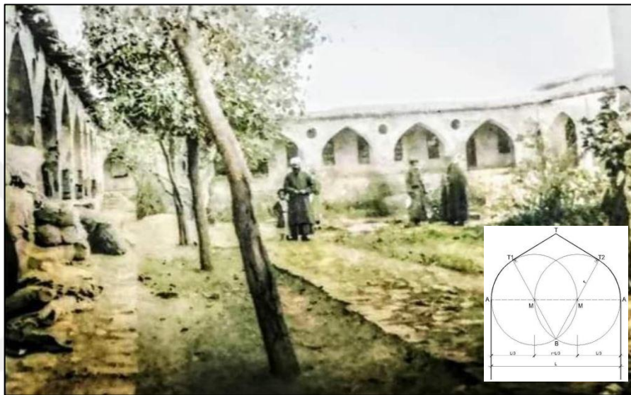
Figure 4.10. Original Turkish pointed arches belong to the Madrasa of the Great Mosque (1900's) before restoration [Anonym].
