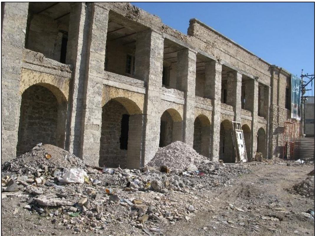
Figure 4.54. Saray during Restoration 2012 [33].
