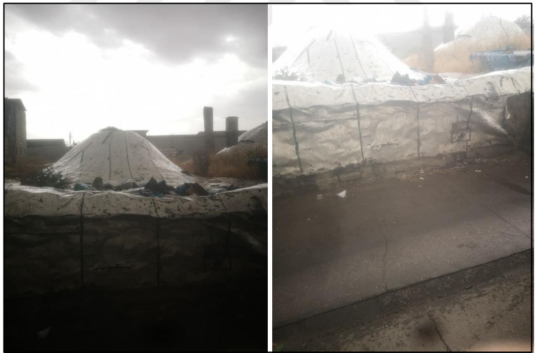
Figure 4.67. Saiwan Hamam's rooftop, photograph taken by author.
