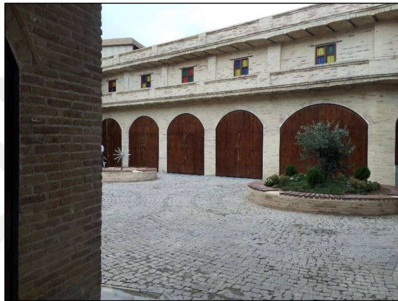
Figure 4.31. Inner courtyard of the Farah Hotel after restoration 2021, photograph taken by author.
