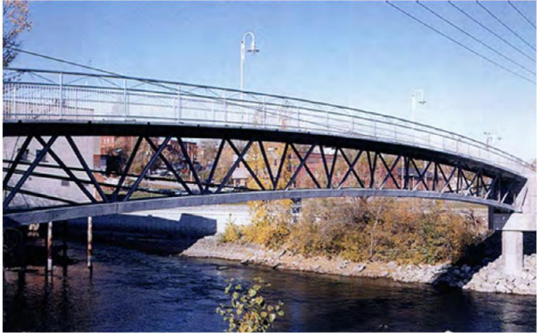
Figure 2.5 Sherbrooke Overpass, the world's first reactive powder concrete bridge (Blais & Couture, 1999)
