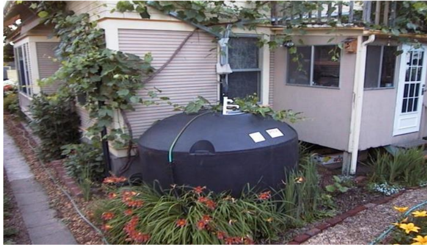
Figure 23. Example of above ground storage (Anonymous 6, 2024)
