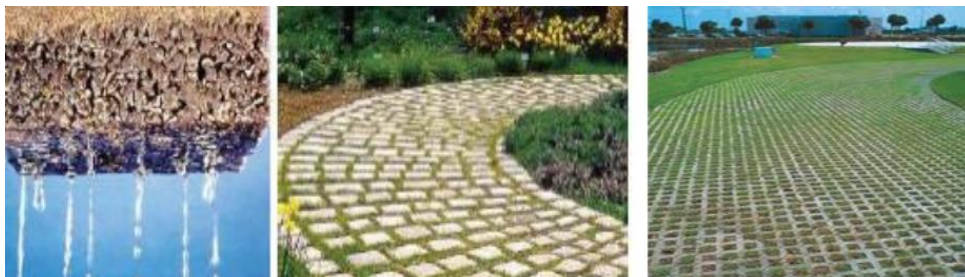
Figure 24. High permeability stones (Tanık, 2017)
