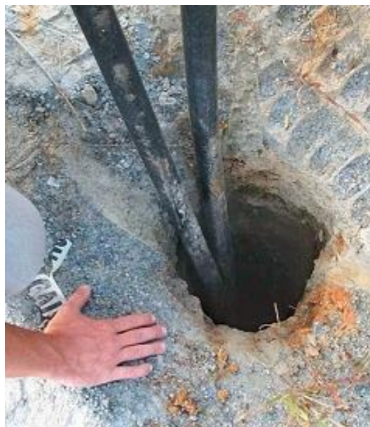
Figure 3.4 : Insertion of vertical U-tube piping prior to backfilling or grouting.
