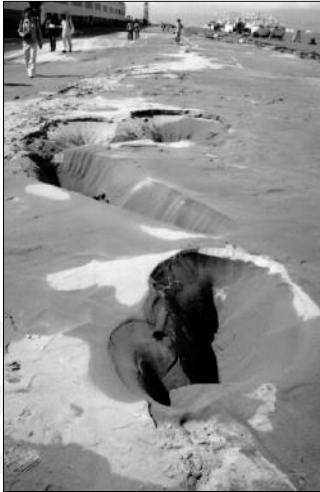
Figure 2.16 The sand boiling due to liquefaction at Hakodate Port, Japan (PIANC, 2001)
