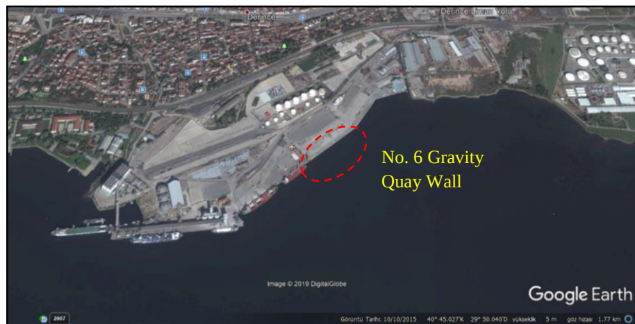
Figure 4.2 Gravity type quay wall inside the Derince Port
