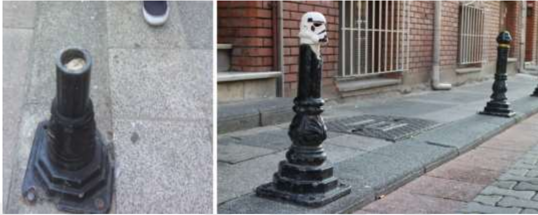
Figure 4.15 Barge without its top components (left), 3D printed heads to replace broken components of barges by P13 and members of Association C (right).
