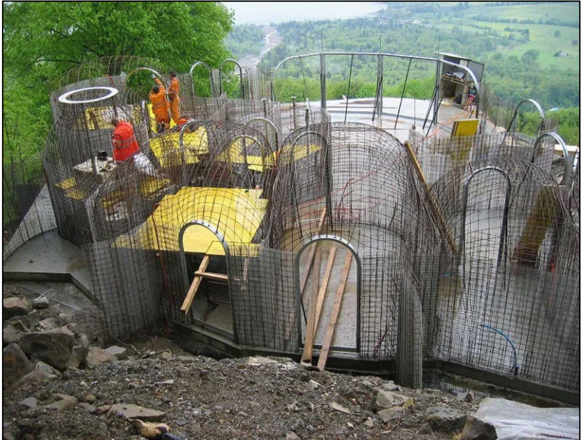
Figure 4.10. Earth House Estate Lättenstrasse House under construction – Switzerland [54].
