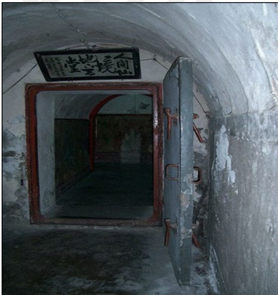
Figure 4.2. Tunnel of Dixia Cheng Underground City [51].
