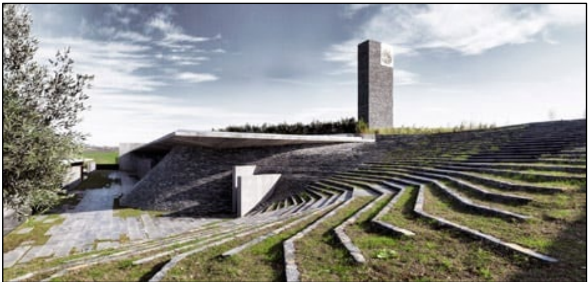
Figure 4.8. Ground-integrated facade of Sancaklar Mosque – Istanbul [53].
