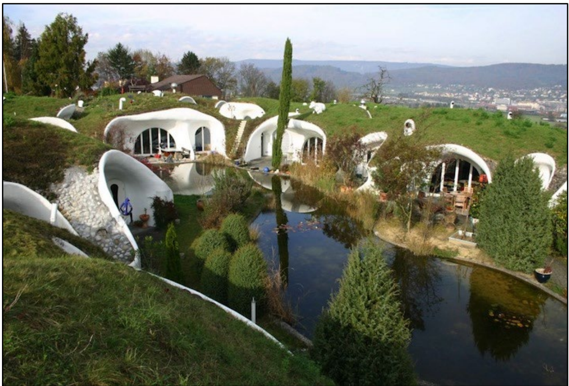
Figure 4.9. Earth House Estate Lättenstrasse – Switzerland [55].
