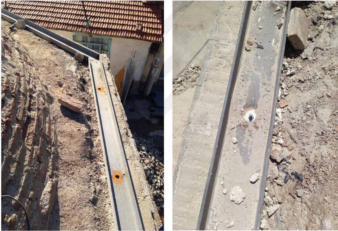
Figure 2.18. Single bar U160 steel girder at the top section of the drum and anchorage connection
