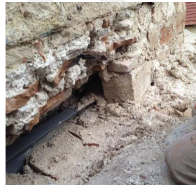
(c) Hydraulic lime based mortar injection and covering
