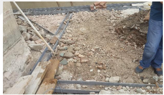
(d) Connection between members
