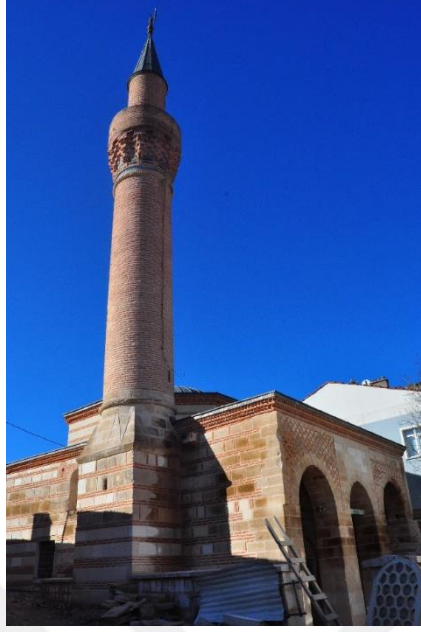
(a) North-East façade
