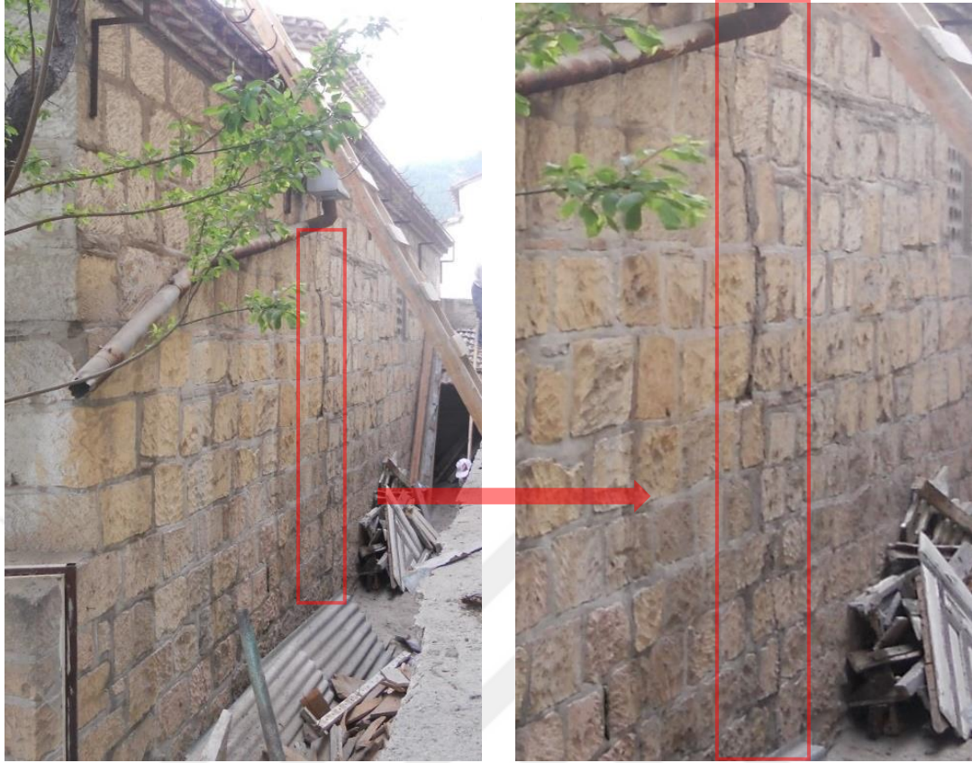
(a) West façade
