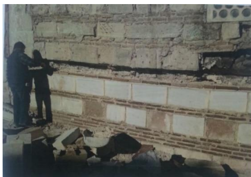
(b) Material decay on the wooden beam located in the South Wall
