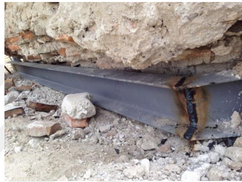
(b) Welded connection
