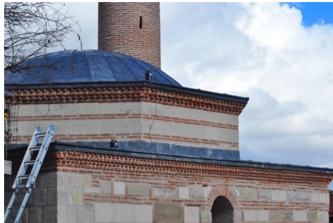
Figure 2.20. Lead covering after steel girder retrofitting
