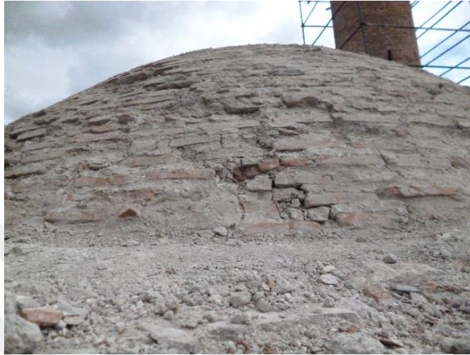
(a) Crack observed on the extrados
