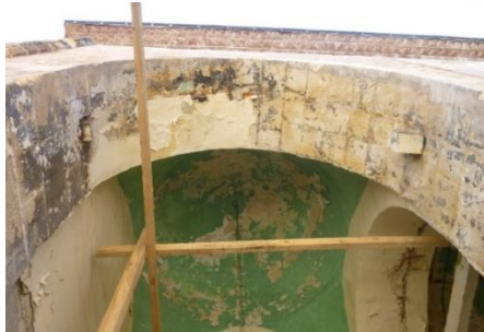
(a) Removed wooden tie beam
