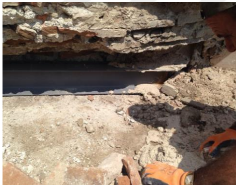
(c) Hydraulic lime based mortar injection and covering
