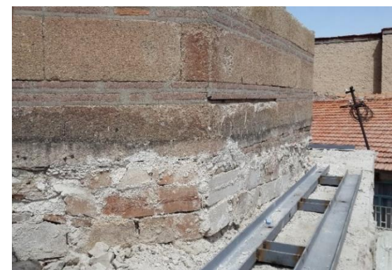
(d) Covering the girders with new masonry material
