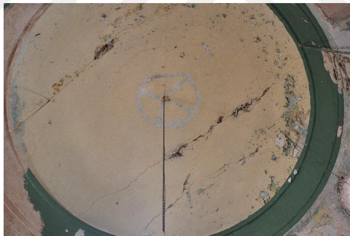
(a) Crack observed on the extrados
