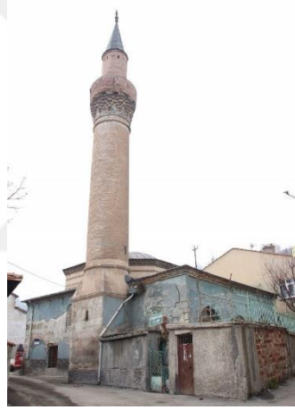
(a) North-East façade (Http-8)
