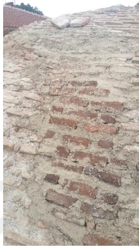
(e) Covering the steel elements
