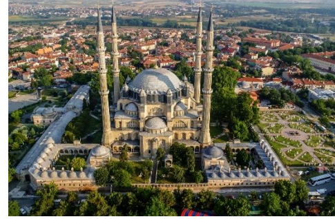
(b) Selimiye Mosque and its Social Complex
