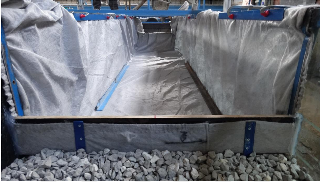
Figure 3.6. Geotextile cover application before the cross-section placement
