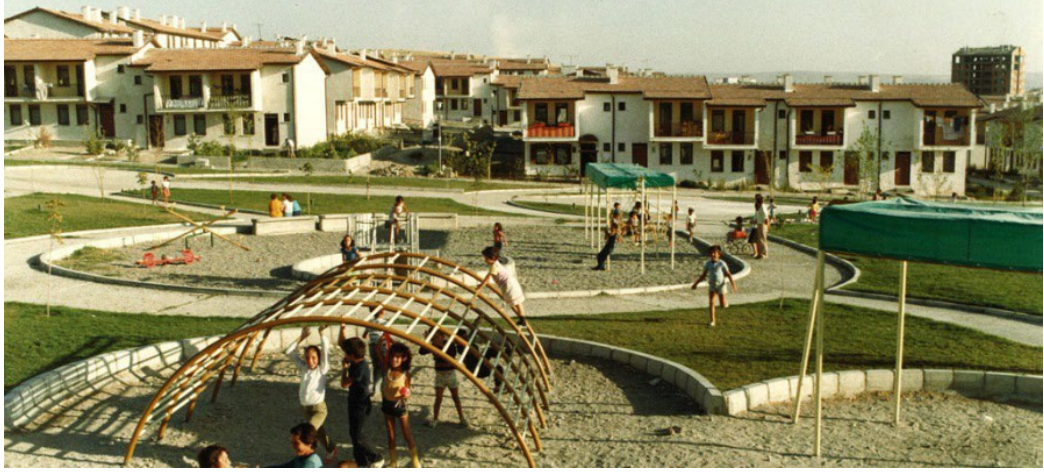
Figure 3. 14 Batıkent Housing Project in Ankara, 1986 (Batikent Project, Ankara - World Habitat, 2018)
