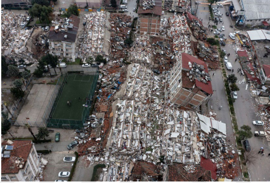
Figure 3. 15 Aftermath of Kahramanmaraş earthquake, 2023 (Medyascope, 2023)
