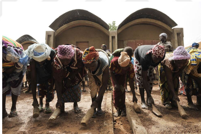
Figure 3. 9 Villagers during the construction ("Kéré | Work" 2023)
