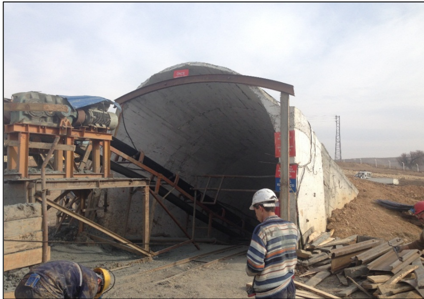
Figure 5.1 : Gallery entrance located in Amasya Suluova Mine
