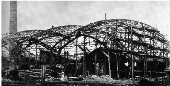
Şekil 3.6 Diagrid formu Exhibit Pavillion, Rusya [21]
