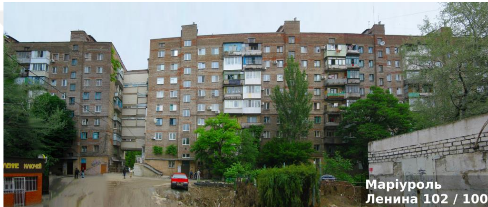
Figure 1.3. Residential structures produced using geopolymer concrete in Ukraine (Hlavacek, 2014).
