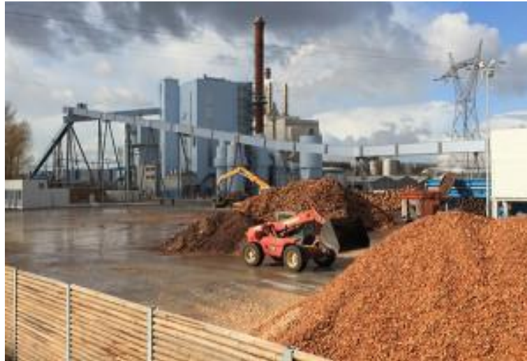
Fig. 1.3. A view from the Pakmil Energy Plant.
