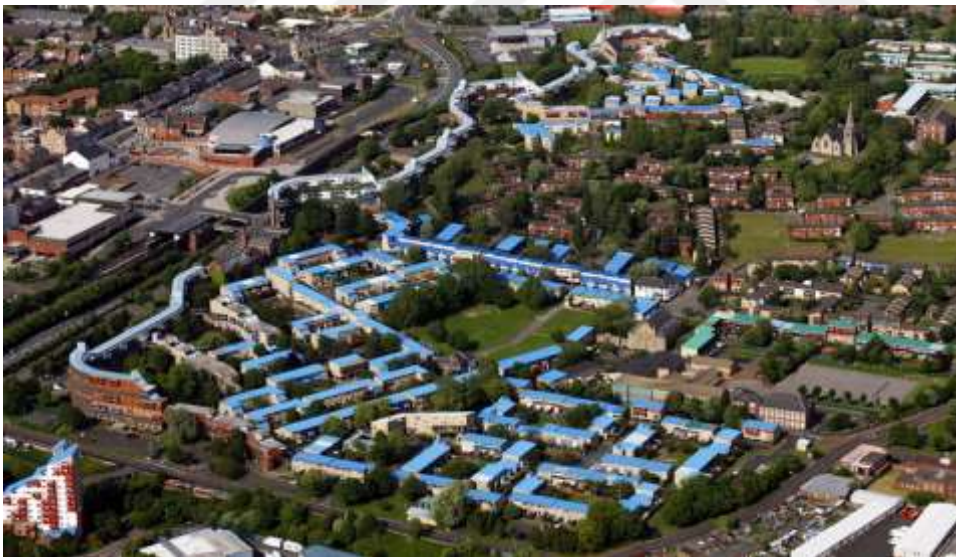
Figure 4.29. Aerial view of Byker housing by Ralph Erskine Source: © Jonathan C.K.Webb. Retrieved from www.webbaviation.co.uk
