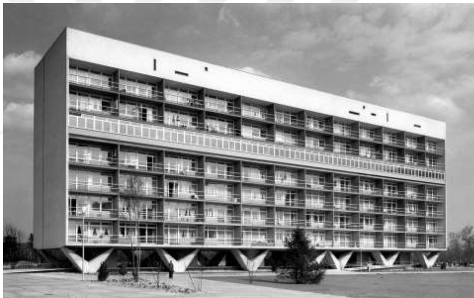
Figure 4.7. Niemeyer Haus by Oscar Niemeyer built in Hansaviertel, Berlin for Interbau (1957)
