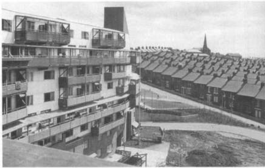
Figure 4.28. The Byker Wall in construction next to the old Byker housing Source: Abrams 2003, p. 121
