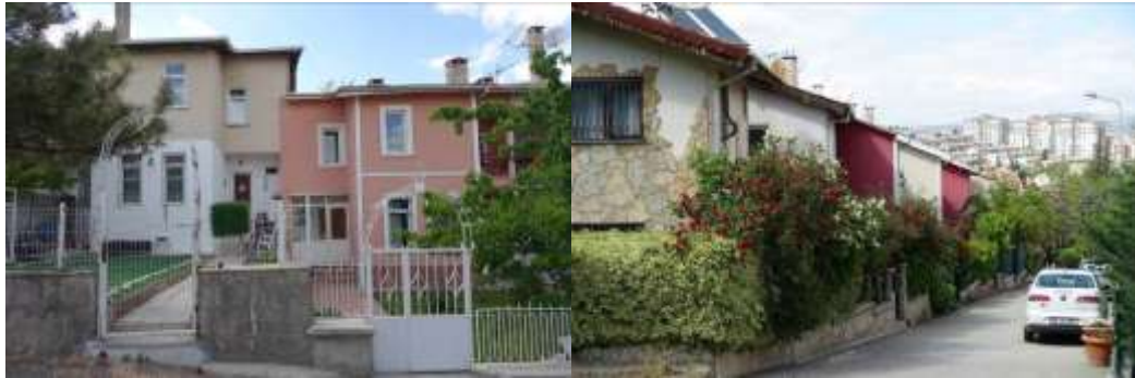
Figure 5.43. Low-density row housing units of Bizim Sokak Sitesi Source: Author
