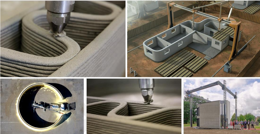
Figure 9: Additive concrete manufacturing process photographs.
