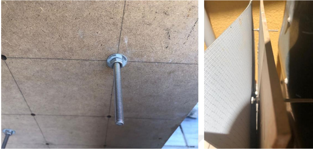
Figure 20: Pin system details. Bolt, nut, and washer combination on the support surface.
