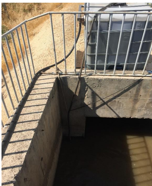
Figure 3.7 Taking wastewater from the influent water of the plant to the first sedimentation tank by pump.
