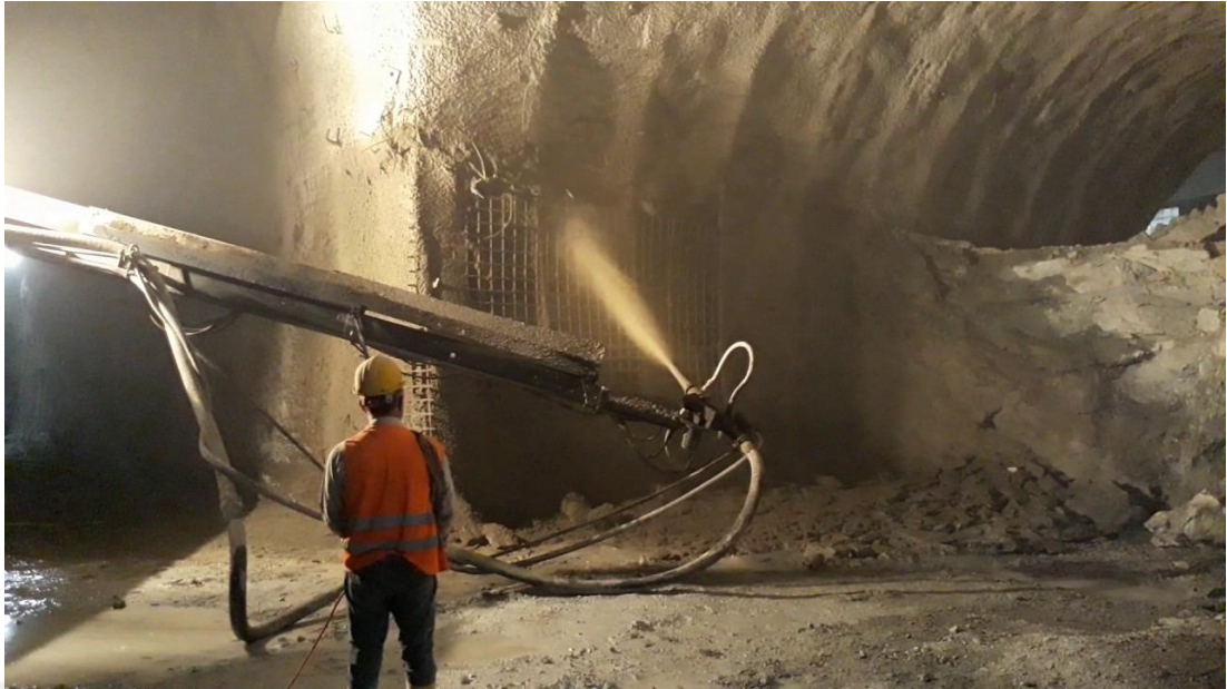
Figure 2.10 In tunnel scotcrete process [11].
