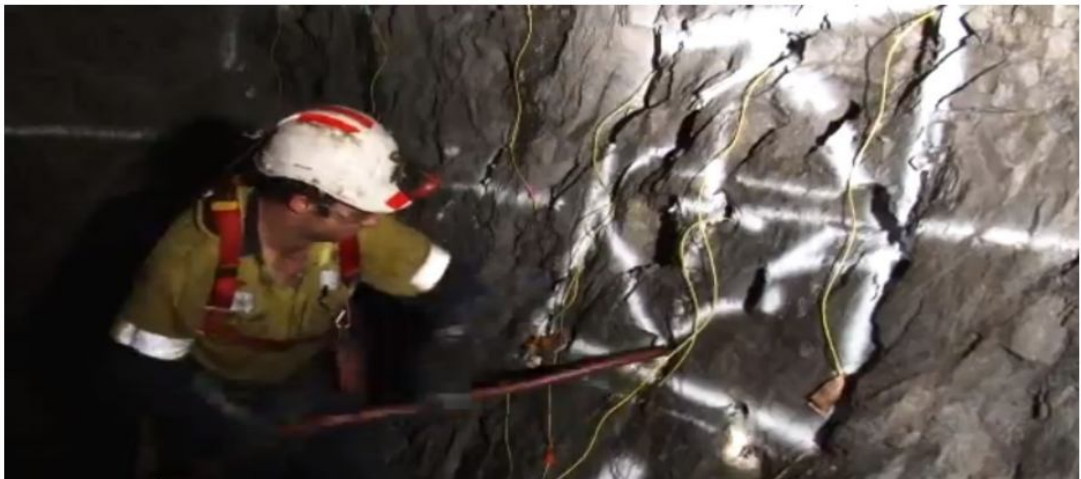
Figure 2.11 Installation of explosives in the tunnel mirror [11].
