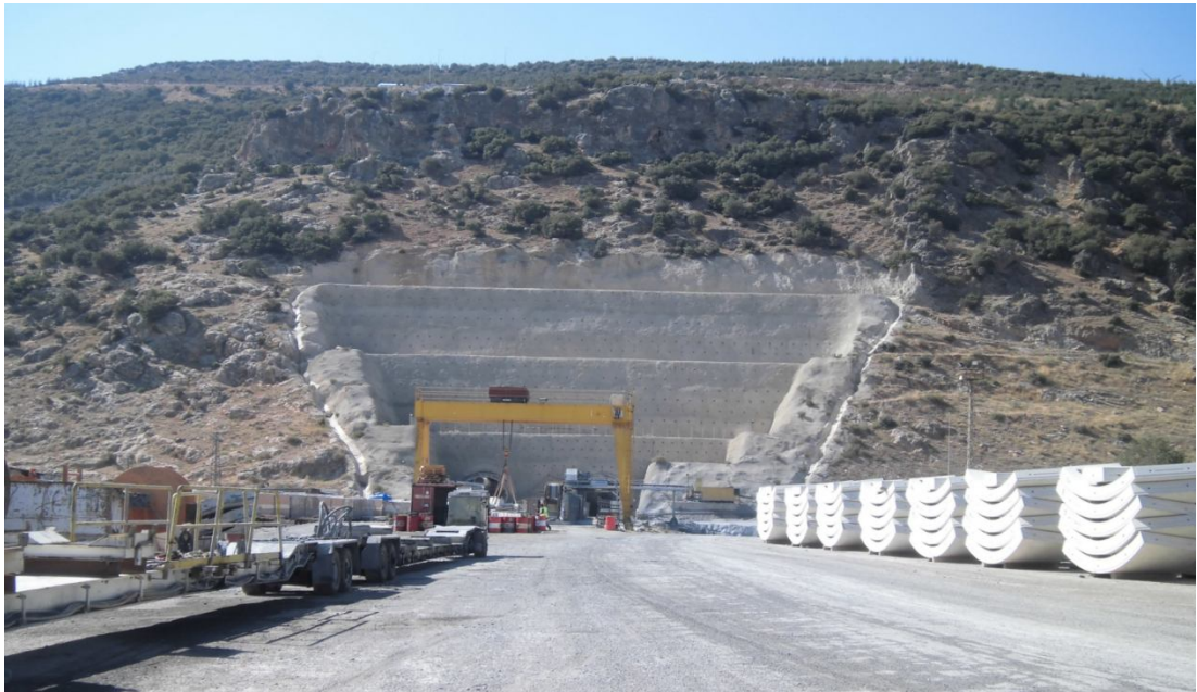
Figure 2.1 Bahçe-Nurdağı tunnel overview (By Musa BUDAK).
