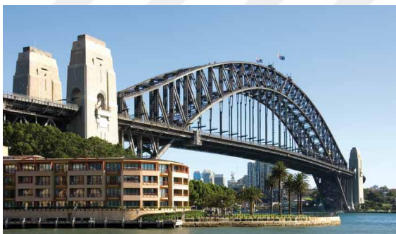
Sydney Harbor Bridge
