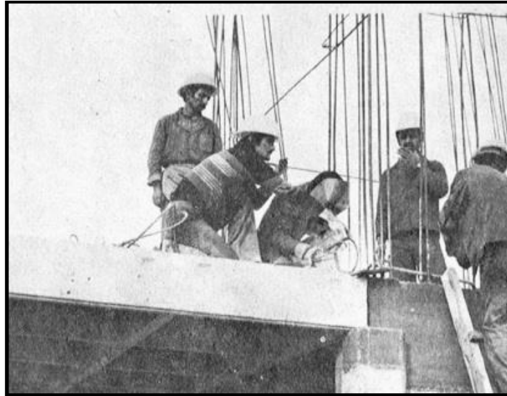
Figure 5.19: The connection of the prefabricated floor slab and the column. (Source: Bulca, A. (1977). İzmit Yeni Yerleşmeler Projesi. Mimarlık , (2), 62.)
