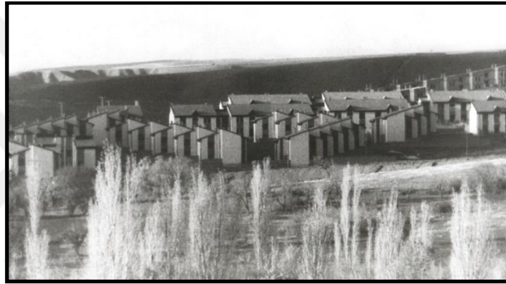
Figure 3.18: A photo from the site, Çorum Binevler Housing Complex. (Source: SALT Research: General Site Photos of Çorum Binevler Housing Complex . [Image]. Retrieved from https://archives.saltresearch.org/handle/123456789/86077 .)
