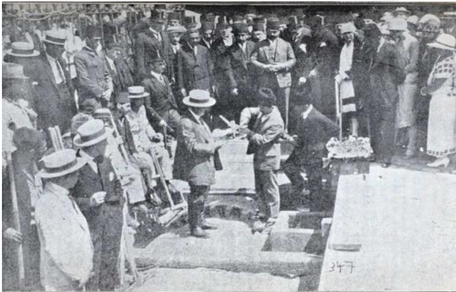
Photograph 3.1 Dr. Emin, who was the mayor of Istanbul, inaugurated the installation of Istanbul's new sewage and drainage system on June 29. SOURCE: Levant Trade Review , vol 13, no 7, (July 1925).
