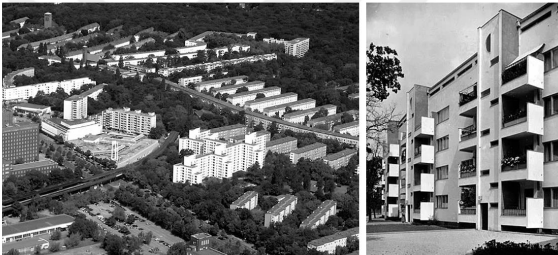
Figure 2.11 Siemensstadt's aerial view and apartment block. (Source: Sharp, D. (1991). Twentieth century architecture : a visual history . Facts on File.)
